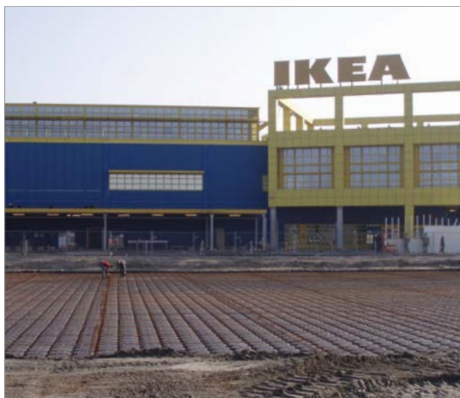
Rainwater dispersion tank under a parking area
