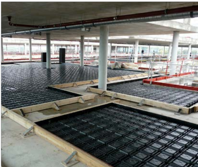
Raising of intermediate floors for office building
