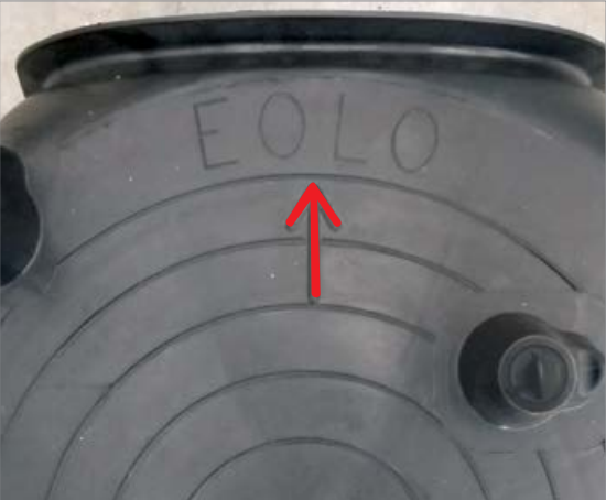
Fig. 1 - Dry positioning of the first formwork, the arrow is facing the foundation curb.
