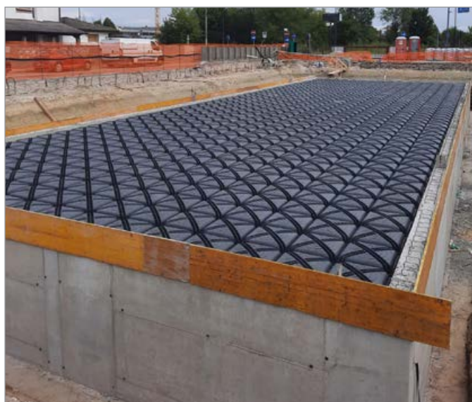
Water collection tank under an industrial area
