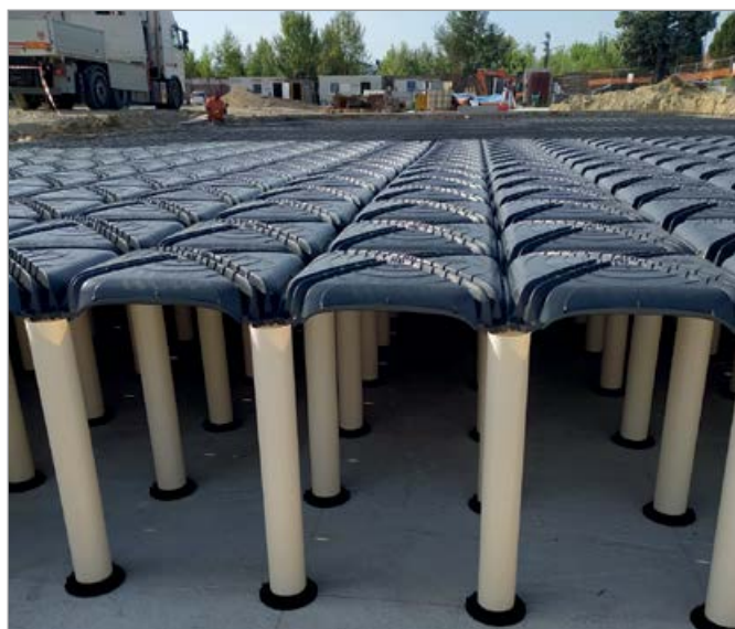
Water collection tank under an industrial area
