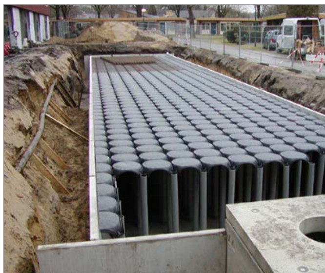
Water dispersion tank under a residential area
