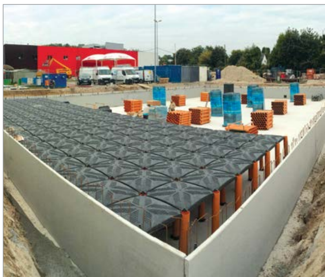
Water collection tank under an industrial area
