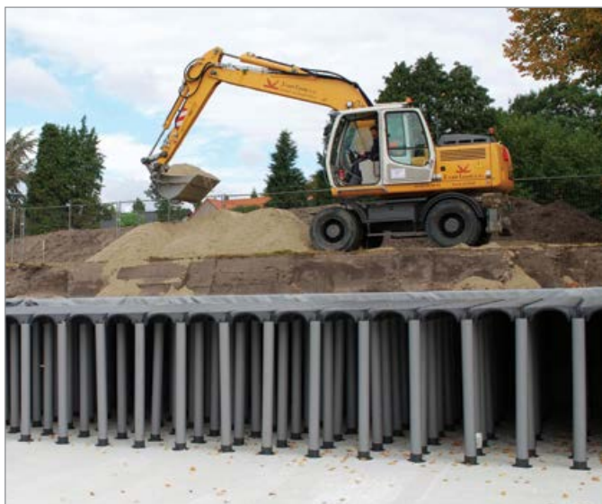
Water dispersion tank under a residential area
