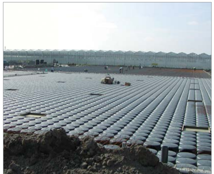
Water collection tank in a greenhouse
