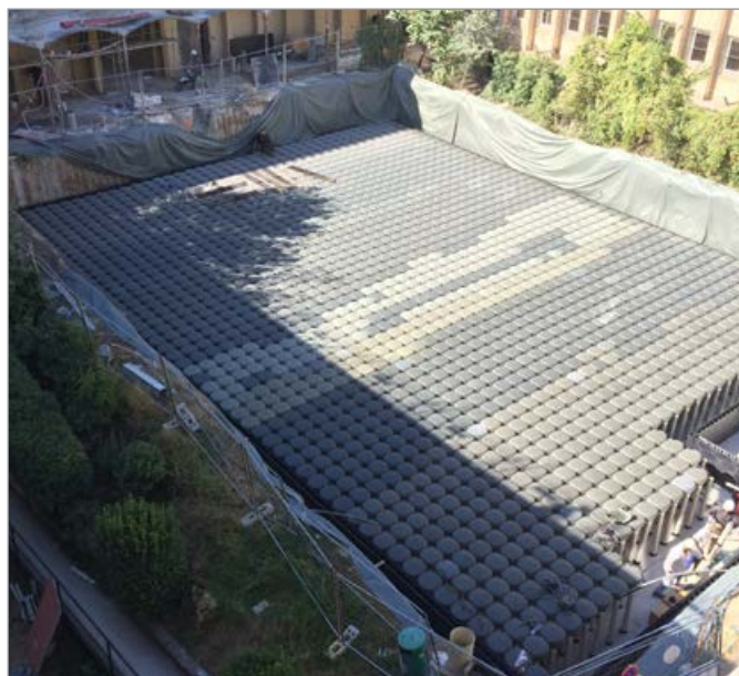
Water collection tank under a residential area
