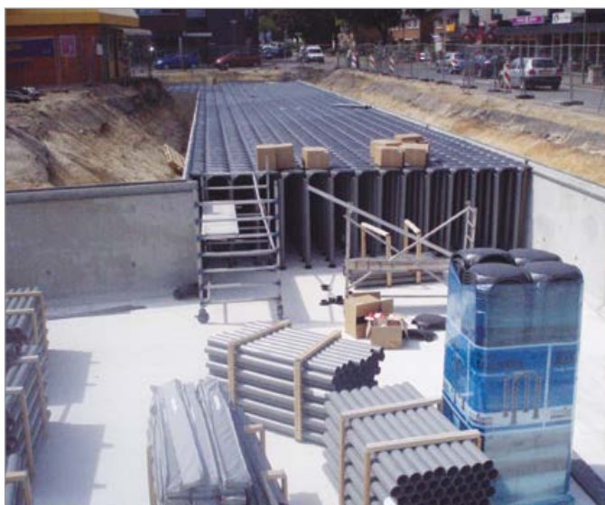
Water collection tank under a commercial parking lot
