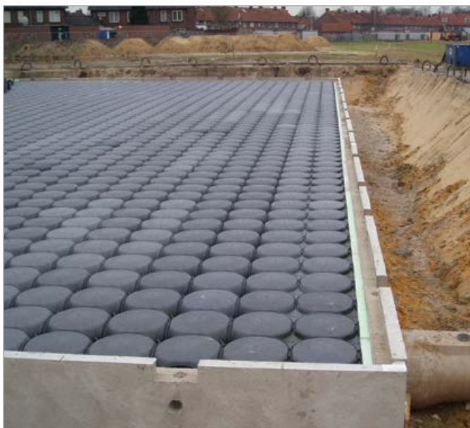
Water collection tank under a green area
