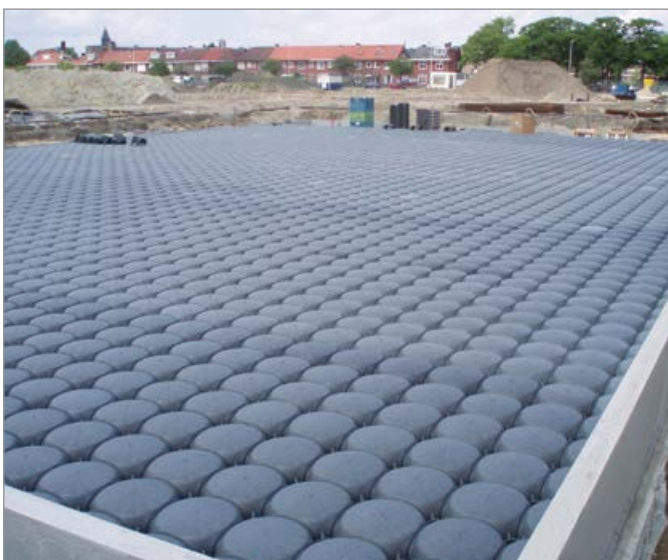
Water collection tank under an industrial area
