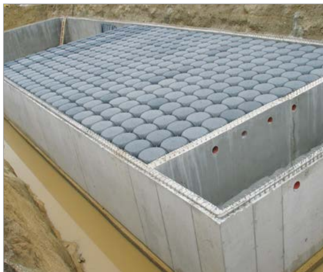
Water collection tank under an industrial area
