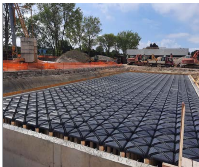
Water collection tank under an industrial area
