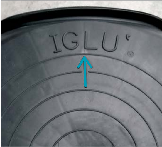
Fig. 1 - Dry positioning of the first formwork, the arrow is facing the foundation curb.
