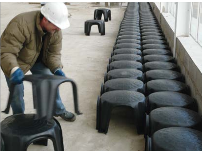
Fig. 3 - Detailed view of the male-female system linking phase - note the perfect seal of the feet.
