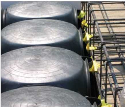
4 After assembling the first Atlantis formworks, position the intermediate stirrups on the panel and then connect the stirrups and collars of the opposing pillars with the steel forks (to be prepared in the construction site).
