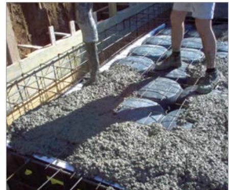
6 Start casting the concrete starting from the pillars, continuing with the curbs and the slab.
