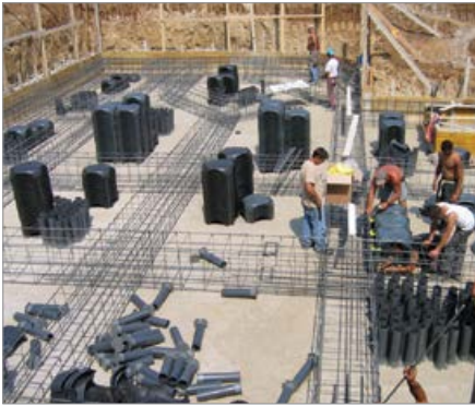
1 Placing the foundation reinforcements on the prepared light concrete base.
