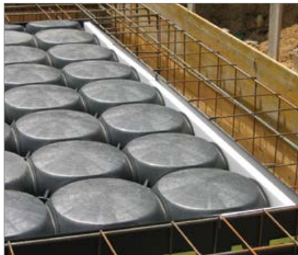
5 Position other panels on top, always fastening them with stirrups and collars, based on the necessary height to be reached. Complete assembling the Atlantis modules and plugging up the side that remained open in the formwork along the perimeter with polystyrene panels.
