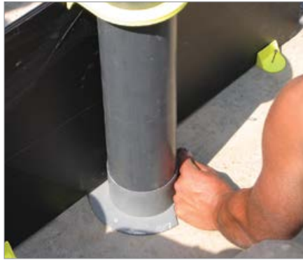
2 Nailing along the inner and perimetric foundation beams of the lower stirrups and pipe base at an equal distance, approx. every 50 cm.
