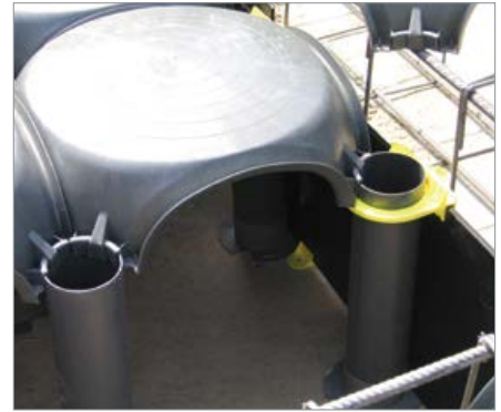
3 Place the initial panel by inserting it in the guide of the lower stirrups and fasten it on the top with the collars inserted on the pillars.
