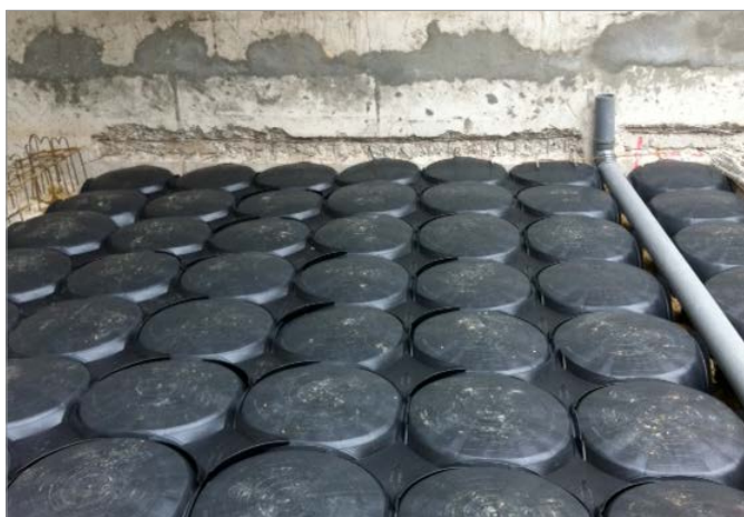
Coffrargile and Beton Up installation
