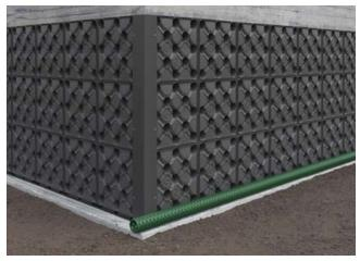
Place the draining pipe along the building perimeter, close to the wall.
