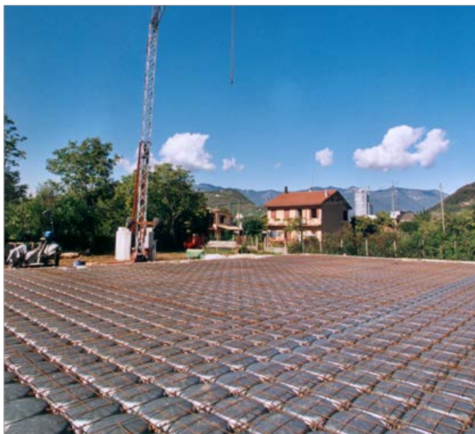
Ventilated under-floor cavity for a building for residential use
