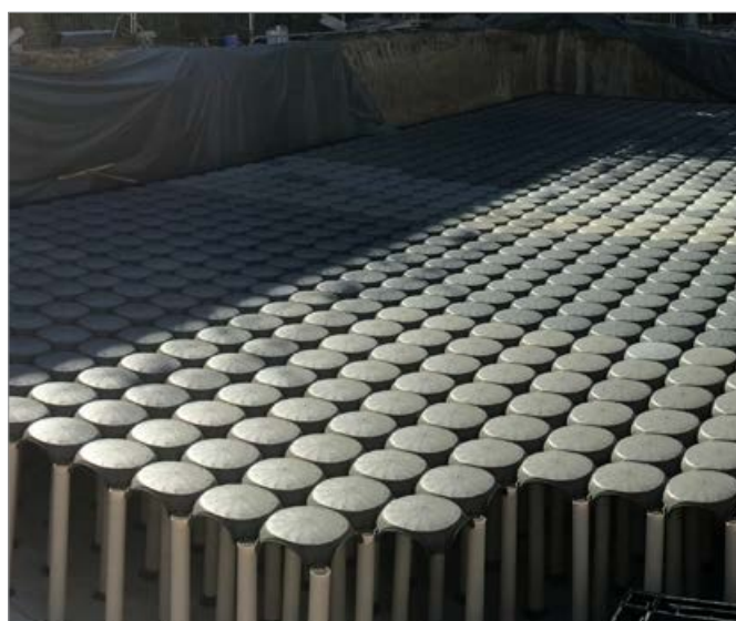
Rainwater accumulation tank
