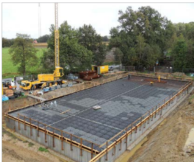
Rainwater accumulation tank
