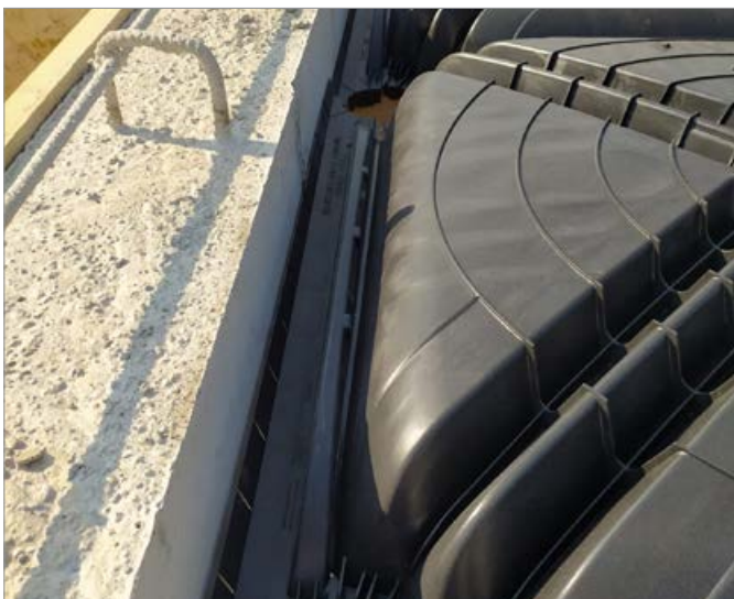
Perfect lateral occlusion thanks to the accessories
