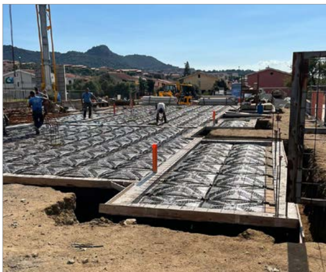
Ventilated under-floor cavity for a building for residential use
