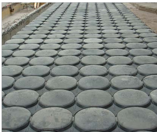
Atlantis system and Beton Up – monolithic slab supported by perimeter
