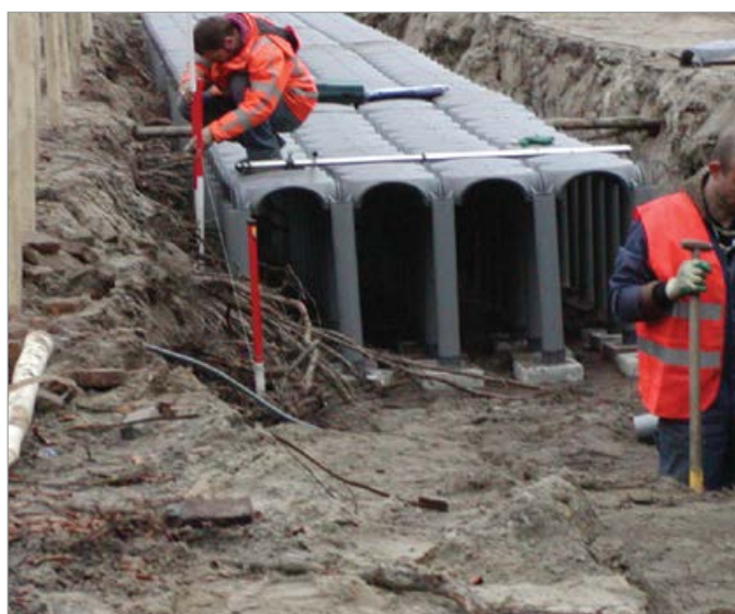
Interspace with root saving function
