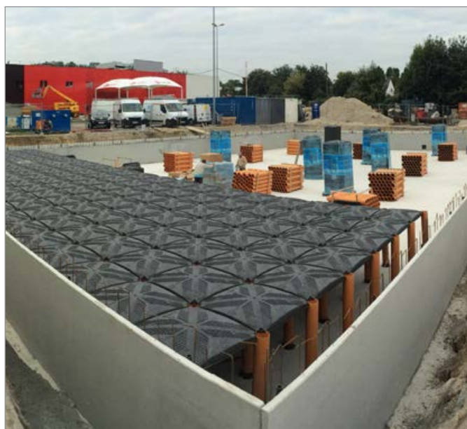
Rainwater accumulation tank under a shopping center
