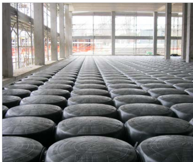
Ventilated cavity for a building for sanitary use
