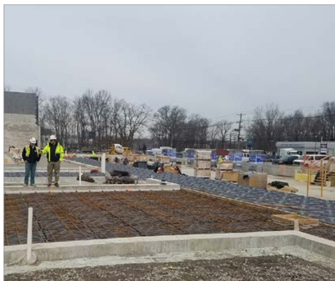
Ventilated under-floor cavity for a building for industrial use
