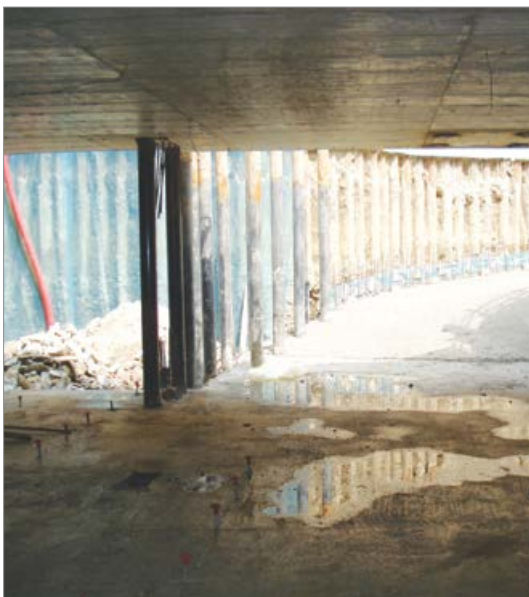
Application example: Underground parking building with the 'top-down' technique.
