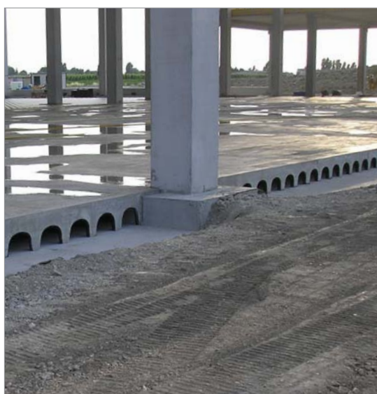
Cella frigo negativa - Alfonsine (RA)
