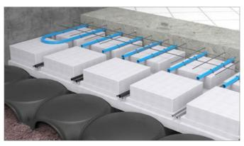
Lay the finishing slab foundation reinforcements and the reinforcements inside the ribbing. Then, cast the concrete in the ribbed slab foundation which should be well beaten down (especially along the sides and in the corners), compacted across its full thickness, supported and trowelled (by hand or using a trowelling machine) to a professional standard. After waiting for the concrete to mature, lay the flooring as per the design.
